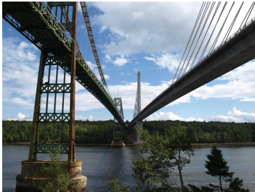
The old and the new bridges at Prospect, Maine (Photo by J. Taggart)
